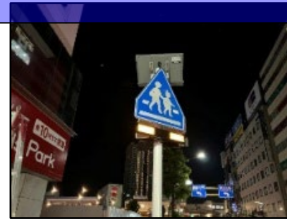
RRFB beacon (Funabashi)
